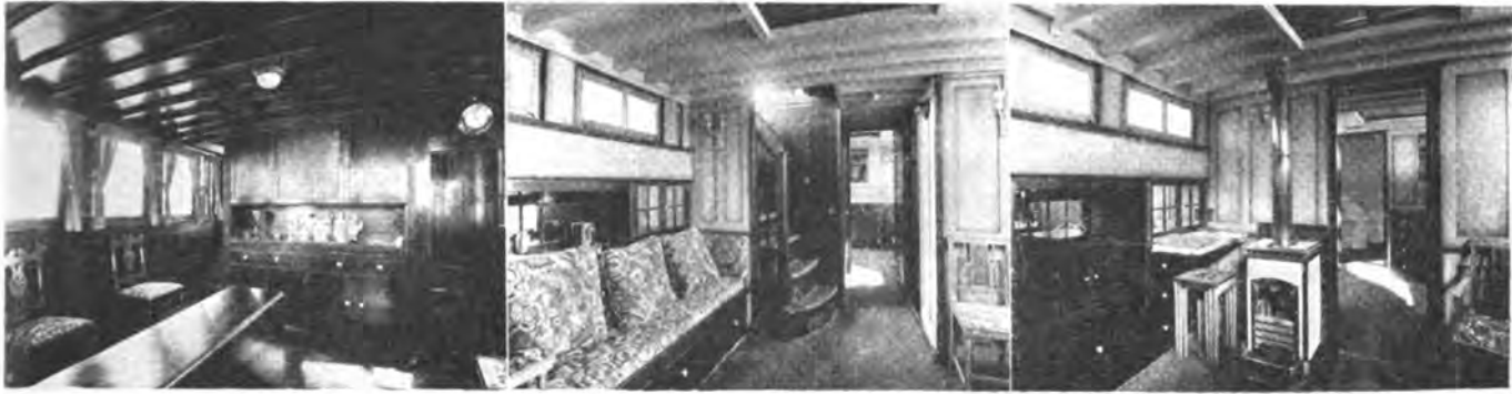
Dining Saloon in the Deck House and Two Views of the Main Saloon Below in Roamer, the New Nock-Designed and Built Yacht for A. Albert Sack, Jr., of Providence. The Furnishings Are in Perfect Taste. Note the Small Tile Stove for Warming the Saloon on Raw Days
