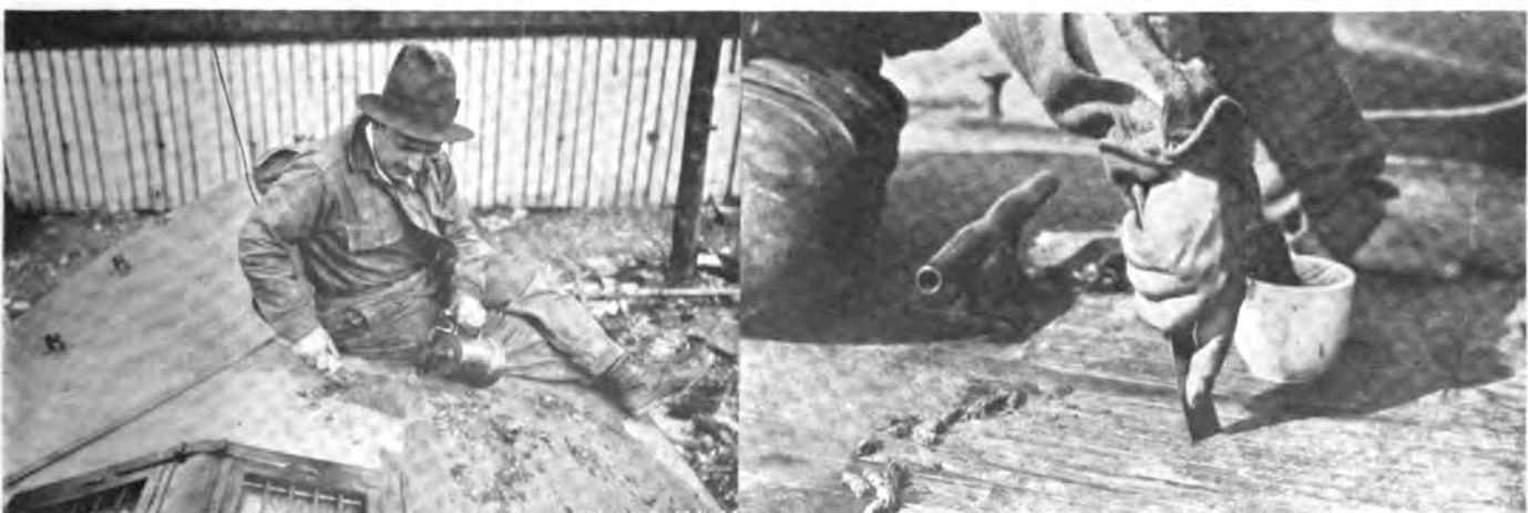
Paint Can be Burned Off a Canvas Deck If You Use Care. If You Use Varnish Remover the Stuff Should Come Off with a Putty Knife
